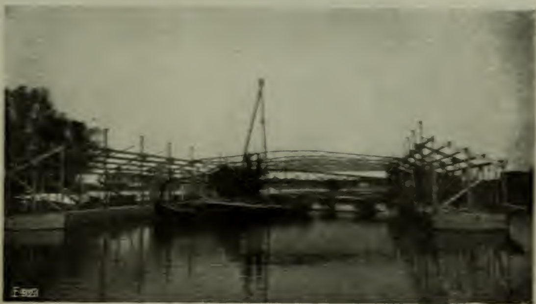
FIG. 3.—BATH DURING ERECTION, SHOWING CONSTRUCTIONAL TIMBERWORK. (See P. 724.)
